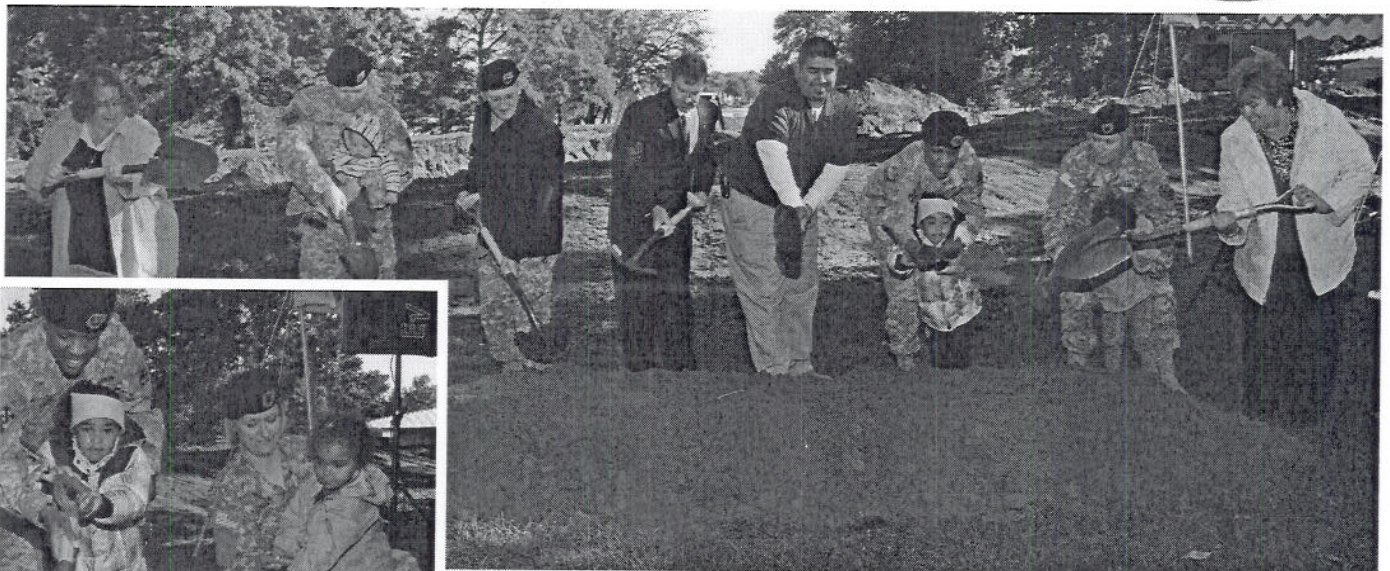
Participants at the ground breaking ceremony toss the first shovels full of dirt to mark the beginning of construction of the new Child Development Center. Pictured above: Kelli Overturf, Rock Island Arsenal Child, Youth & School Services; Maj. Joe Flood, Army Sustainment Command, with his son Sebastian; Maj. Gen. Robert Radin, commander, Army Sustainment Command; Joel Himsl, Garrison Manager; Salvador Murillo, general manager, Murillo Modular Group LTD; Sgt. 1st Class DeShonda Davis-Locke, Army Sustainment Command, with her daughter Kyasue; 1st Lt. Tonda Thomas, Community Based Health Care Organization, with her daughter Tamber, and Debi Behl, Rock Island Arsenal Child, Youth & School Services. Left: Davis-Locke and Thomas give their daughters another shot at the dirt.
